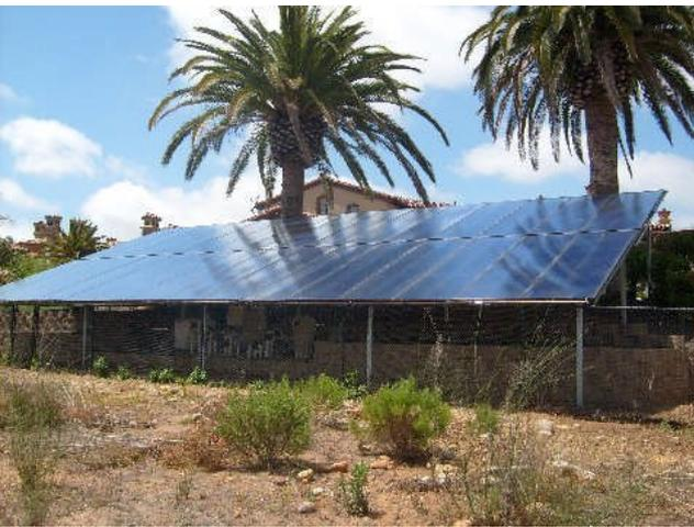
Average percentage of collector area to pool surface area coverage is generally 70% as recommended by the manufacturer. A south facing 50% coverage will generally give one to three additional months of pool usage at each end of the season. Some customers have requested pool systems with as little as 25% coverage with good results for their needs.
